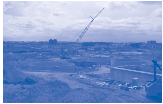
Arapahoe County Water & Wastewater Authority, Lone Tree Creek Water Reuse Facility
